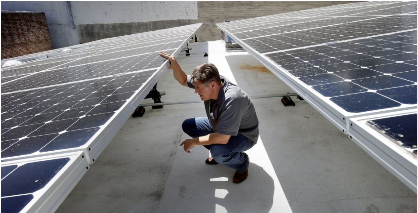
Figure 5. Ted van der Linden, Sustainability Director at DPR Construction, inspecting the PV array on the roof of their newly renovated San Francisco headquarters building. The building has submitted its LEED v4 Platinum certification to the U.S. Green Building Council as well as Net Positive Certified from the International Living Future Institute.
