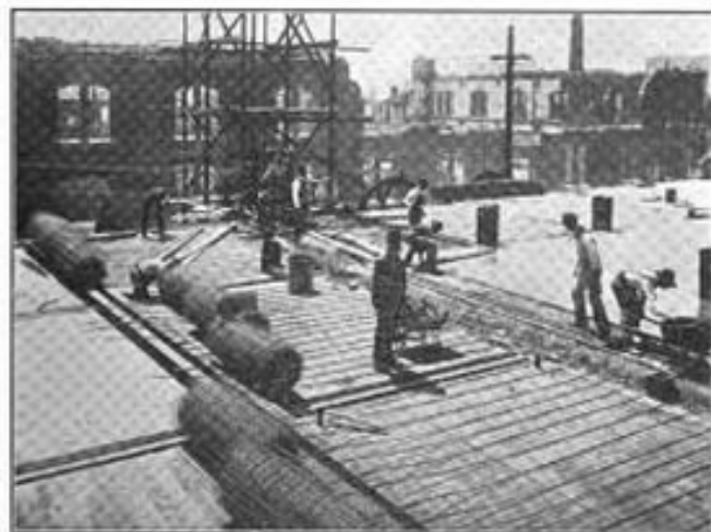
The Plant of A. SCHILLING & CO., Second and Fulton Streets, the first permanent Concrete Building erected after the disaster. American System of Reinforcing used throughout
