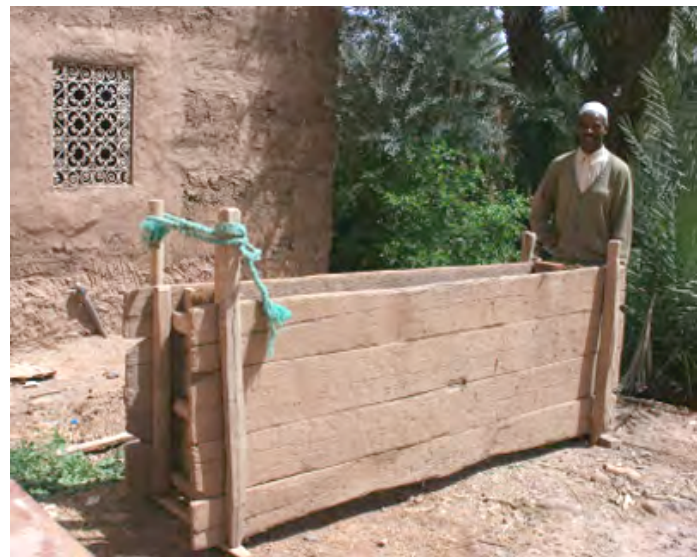
formwork in place around rammed earth wall
